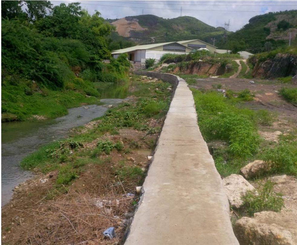
Figure 2: Soil erosion preventive measure at Pangdan
