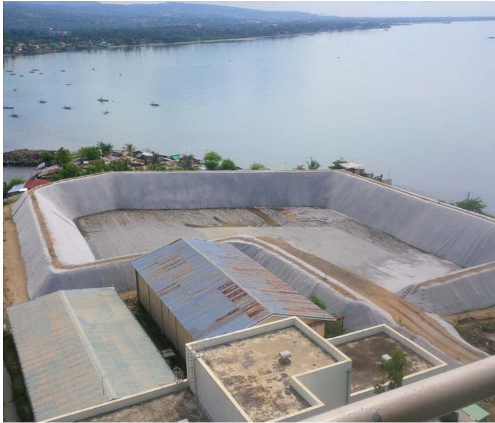
Figure 1: Completed Emergency Ash Pond B at KSPC Compound
